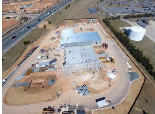
Figure 15: New Station Construction Begins
